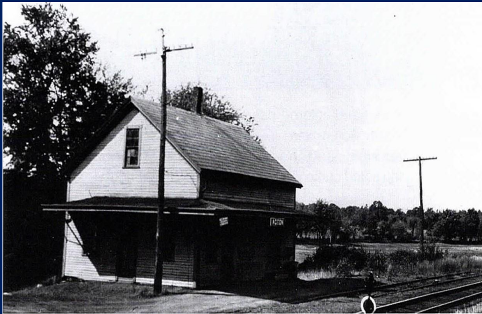
Notice two sets of rails F&L in foreground
